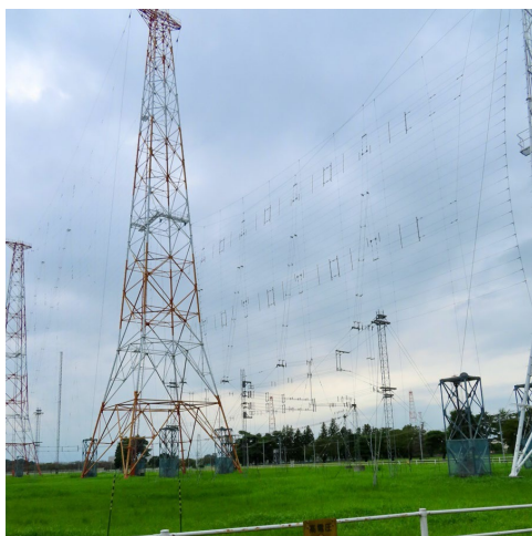
Fig.3 High-performance curtain antenna
