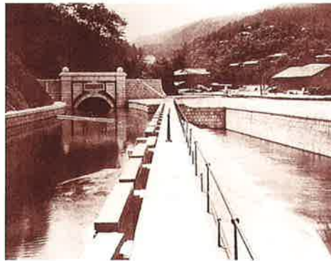
The joint tunnel of the first and second canals, the head tank and the spillway
