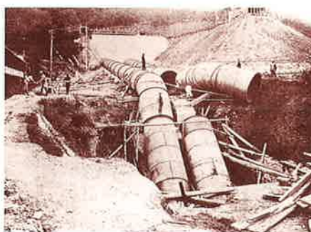
Installation of penstocks
